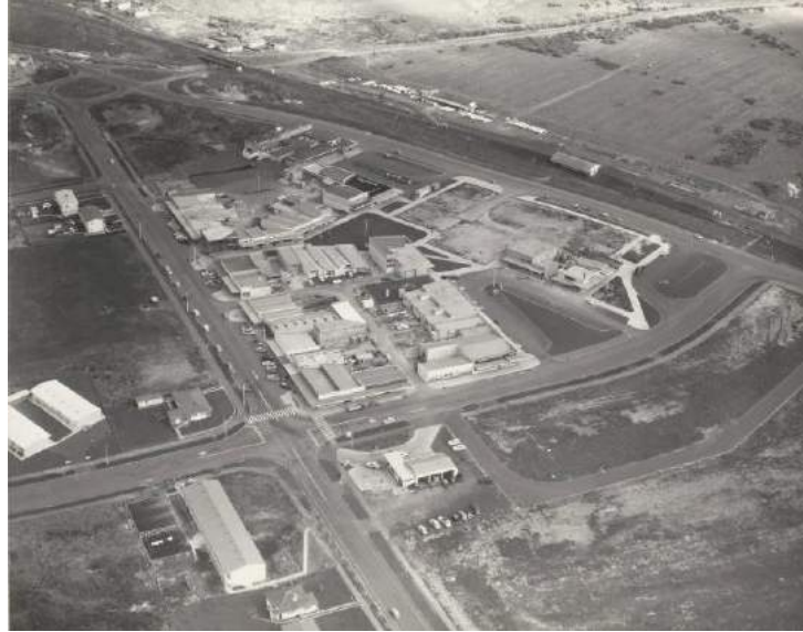
Glen Innes 1960 showing construction of Glen Innes Shopping centre
