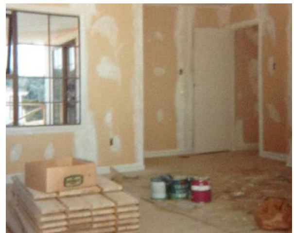
The plastering complete!
