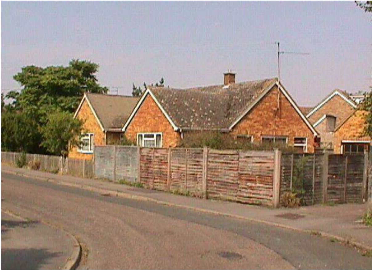
Our home in Oxfordshire - 1 Willow Mead, Chalgrove
