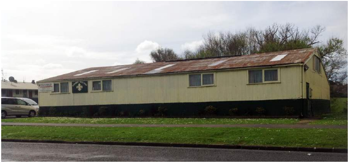
Glen Innes Scout Den, Taniwha Street (now demolished)
